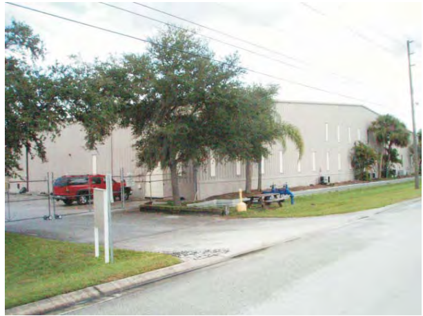
View of the adjacent Roll-A-Way window and shutter to the east
