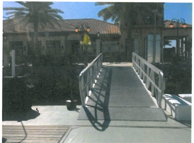
Marina Office and Restaurant
