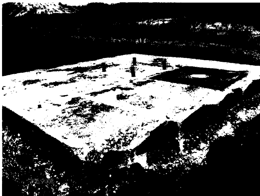
Typical View of a Water Well Foundation
