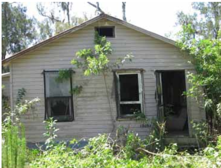
Photo 6.3. North elevation of 13037 Vogel Farms Road (8HI11361), looking south.
