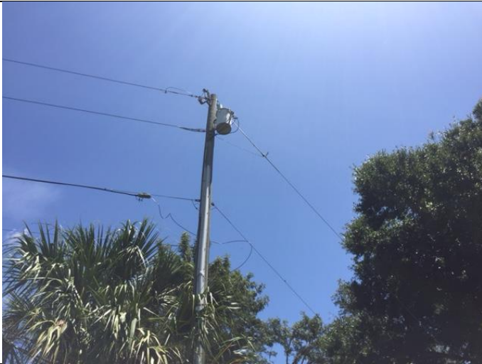
Photograph 11 – View of electrical transformer located along northern boundary of property
